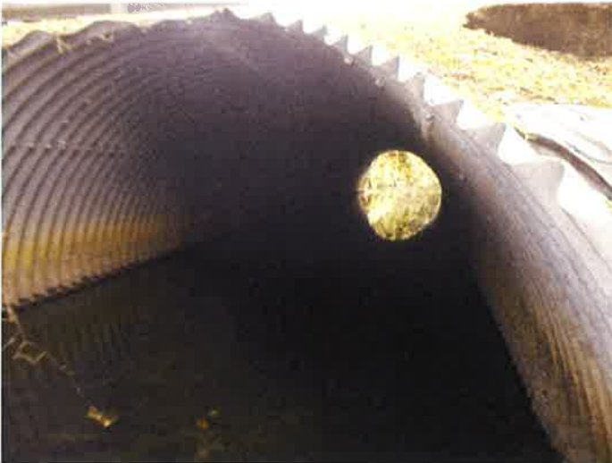
Document Name: DSCN0410.JPG Category: Culvert Comments: West culvert
