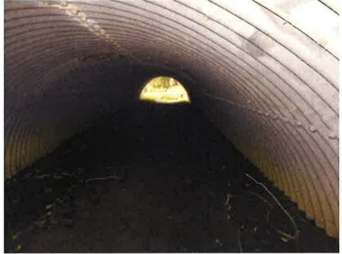
Document Name: DSCN0406.JPG Category: Culvert Comments: East culvert
