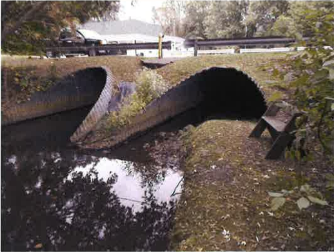
Document Name: DSCN0411.JPG Category: Elevation Comments: South elevation
